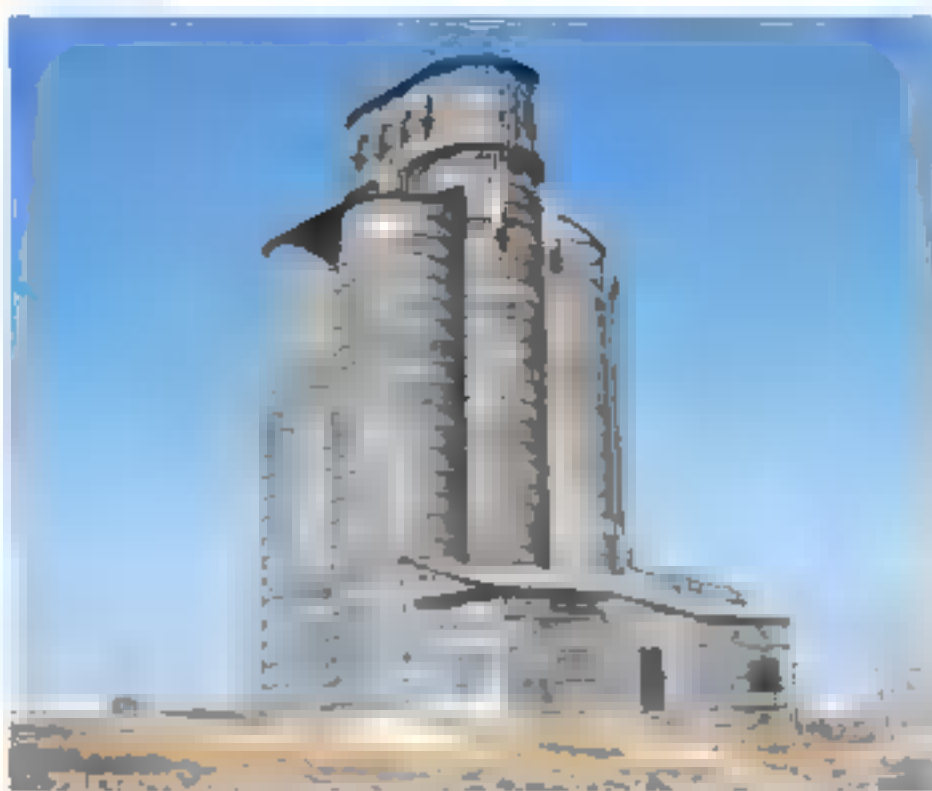
Former sugar silos now hold phone gear.
